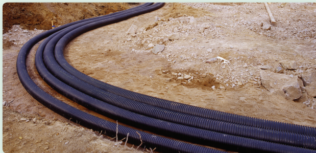
Flexible Ecoflex Pre-insulated Pipe
